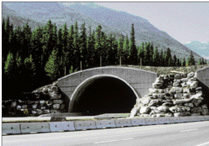
During the twinning of the highway, two experimental wildlife overpasses were built in an effort to counteract the barrier effects of the Trans Canada Highway. Photo: D. Draper.
